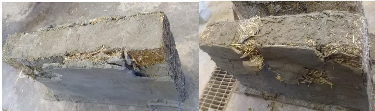
Fig. (6). Failure partner of plastered wall.
